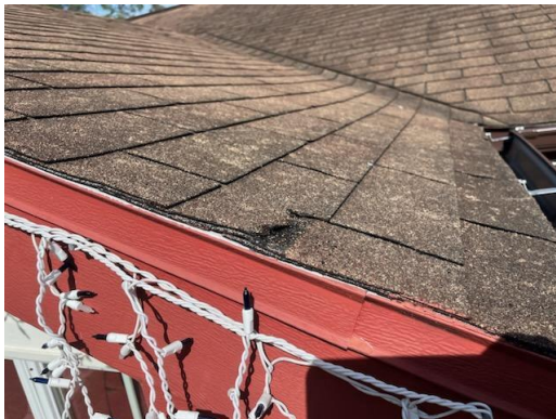
1509-3 Asphalt Shingle Typical Exterior Roof
